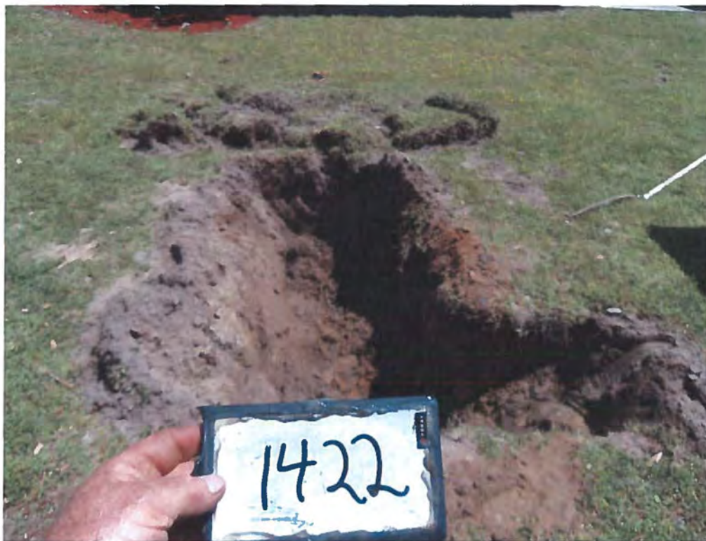
Picture 2: UST 1422 Albatross excavation.
